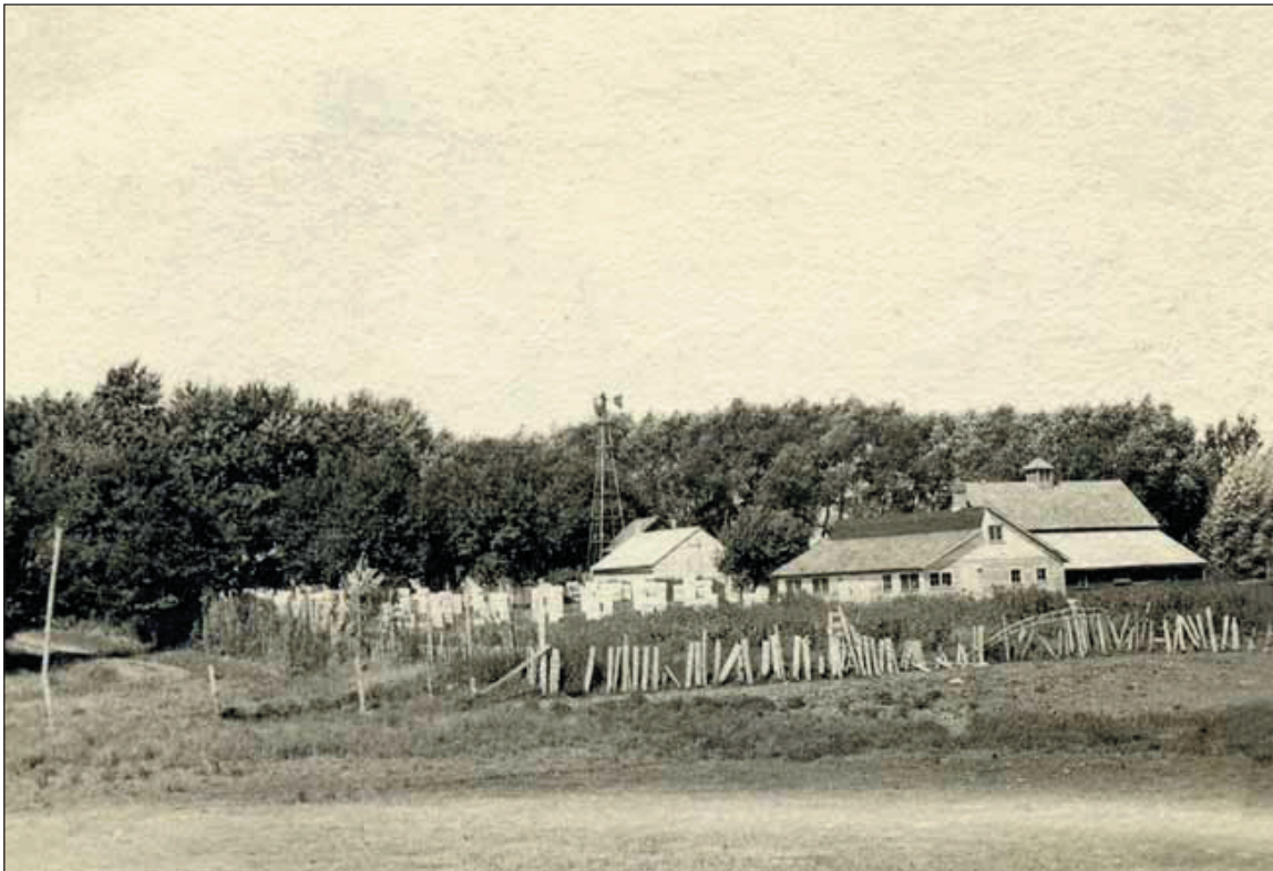
figure 11. View of the south home yard showing a newly constructed bee cellar in which bees were kept during winter. The cellar is the light-colored structure between the honey house and the windmill. For many years all bees were kept in cellars during winter, and at one point there were four cellars: two at the home place and two in out-yards. Photo probably taken sometime between 1915 and 1920.
