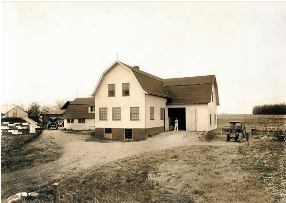
figure 14. The honey house with Emil standing in the garage door opening. This and the next photo appeared in the 1925 March and April issues of American Bee Journal in a two-part article about Emil, his modern facilities and efficient business practices.
